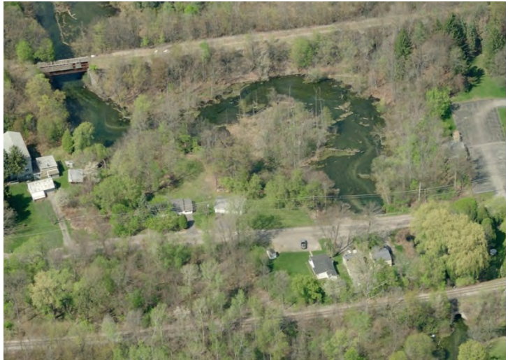
Figure 2 Houses along Mill Street (Land Conservation zone)
