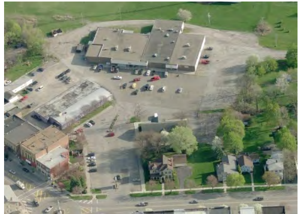
Figure 16 Village parking lot at Caledonia Commons – view from north, 2010 (Source: Pictometry)
