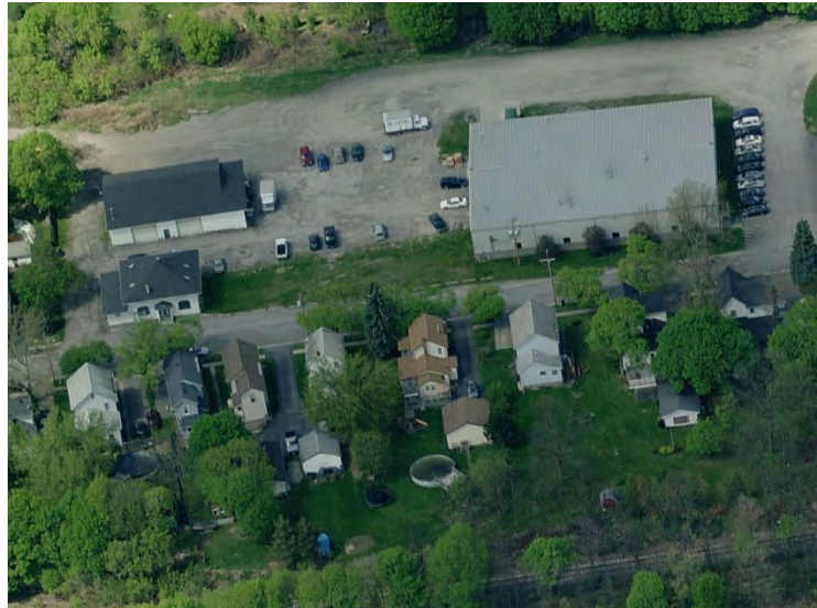
Figure 1 Industrial buildings and houses along Lehigh Street
